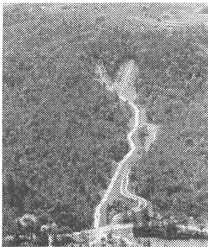
Fig. 2 Aerial photograph of Ikeno-ue landslide after stabilization construction
